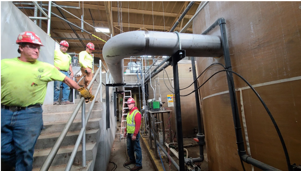
Temporary Gravity Belt Thickener drain tied into new collection tank to be pumped to Grit Chamber.
