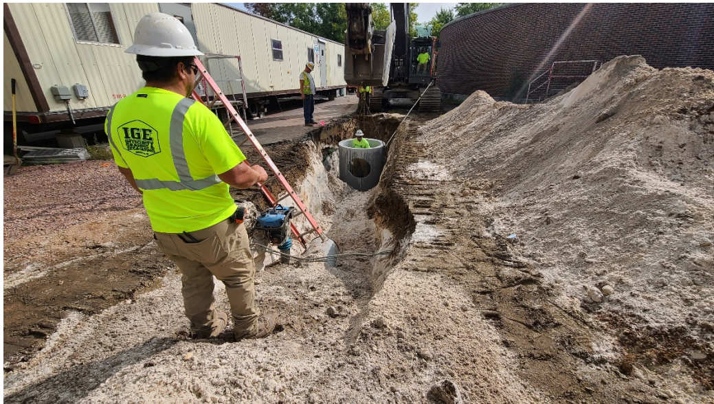
New storm sewer between Structure 110 (Vehicle Storage Building) and Structure 700 (Digester Building) to drain storm water from Structure 100 (Main Building).
