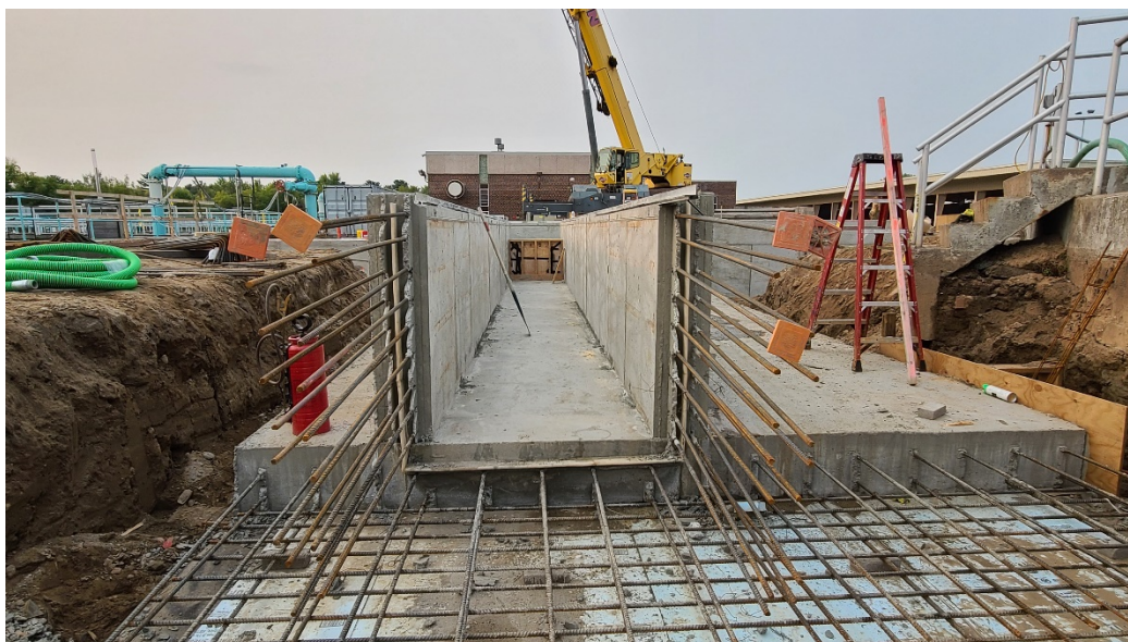
Looking south down new Structure 350 (Primary Effluent Channel).
