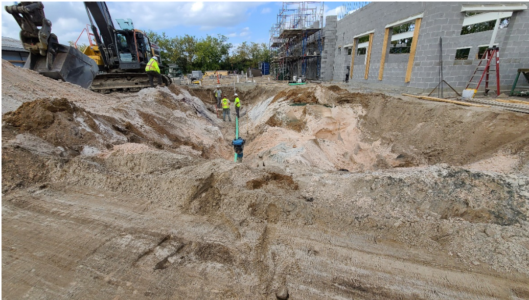
New sanitary sewer connection for Structure 120 (Administration Building).
