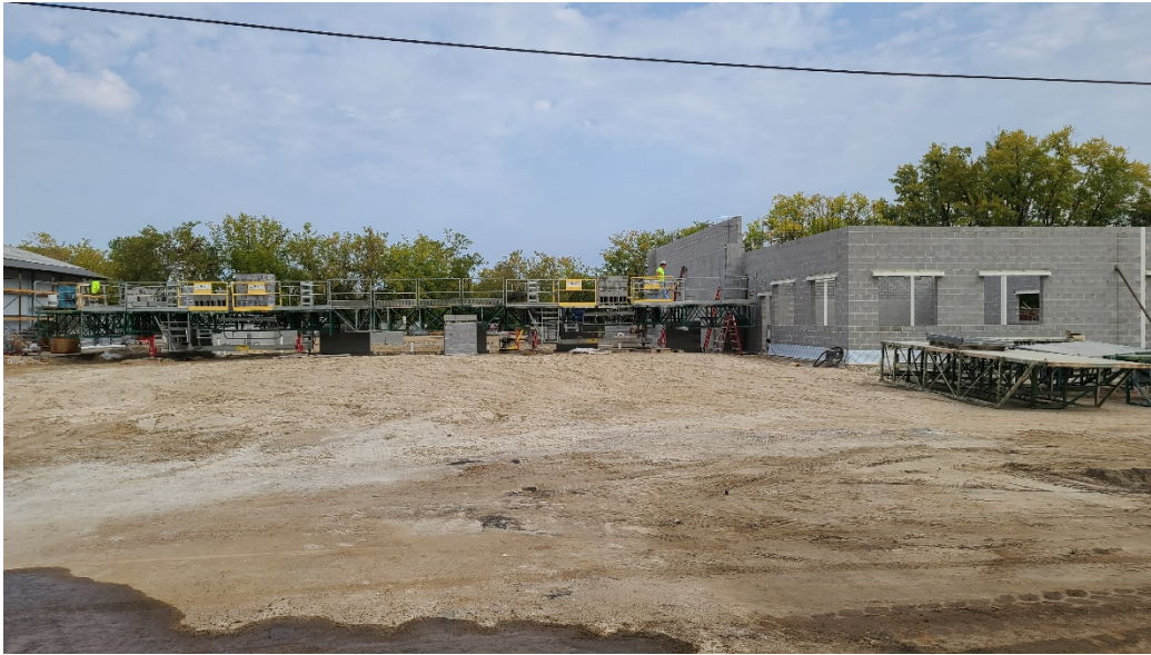
Concrete masonry unit walls going up in garage of Structure 120 (Administration Building)
