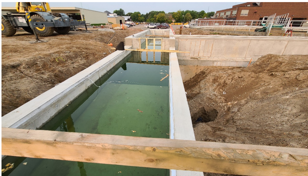
Structure 404 (Junction Structure) water test.
