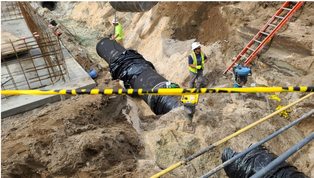
Placing yard piping between new Structure 610 (Chemical Building) and existing Structure 600 (Effluent Building).
