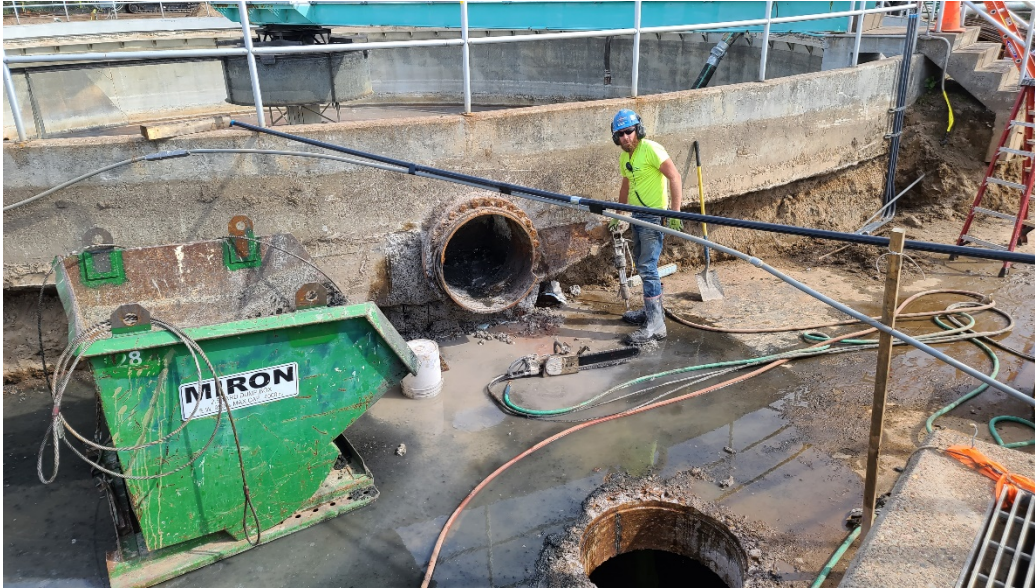
Demolition work has started on Structure 340 (Primary 4) to allow for future tie in to Structure 350 (Primary Effluent Channel).
