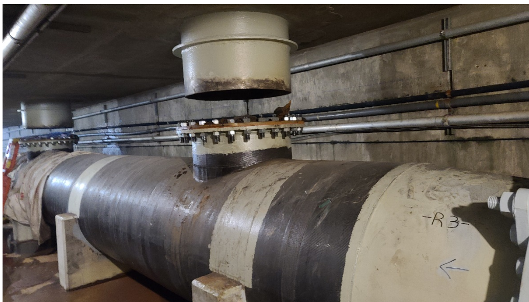
Primary Clarifiers 3 and 4 disconnected from existing primary effluent piping.
