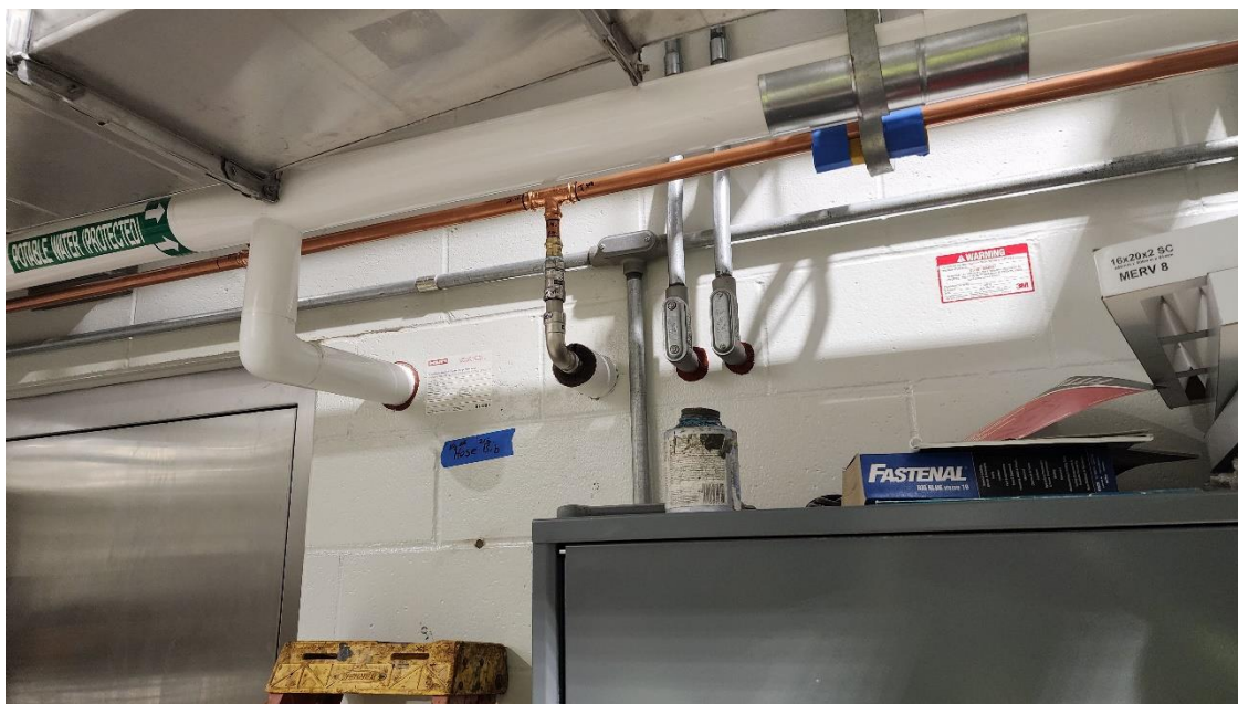
New Hot Water Line feed to each chemical room for the ability of a hot water wash down in Structure 100 (Process Building).
