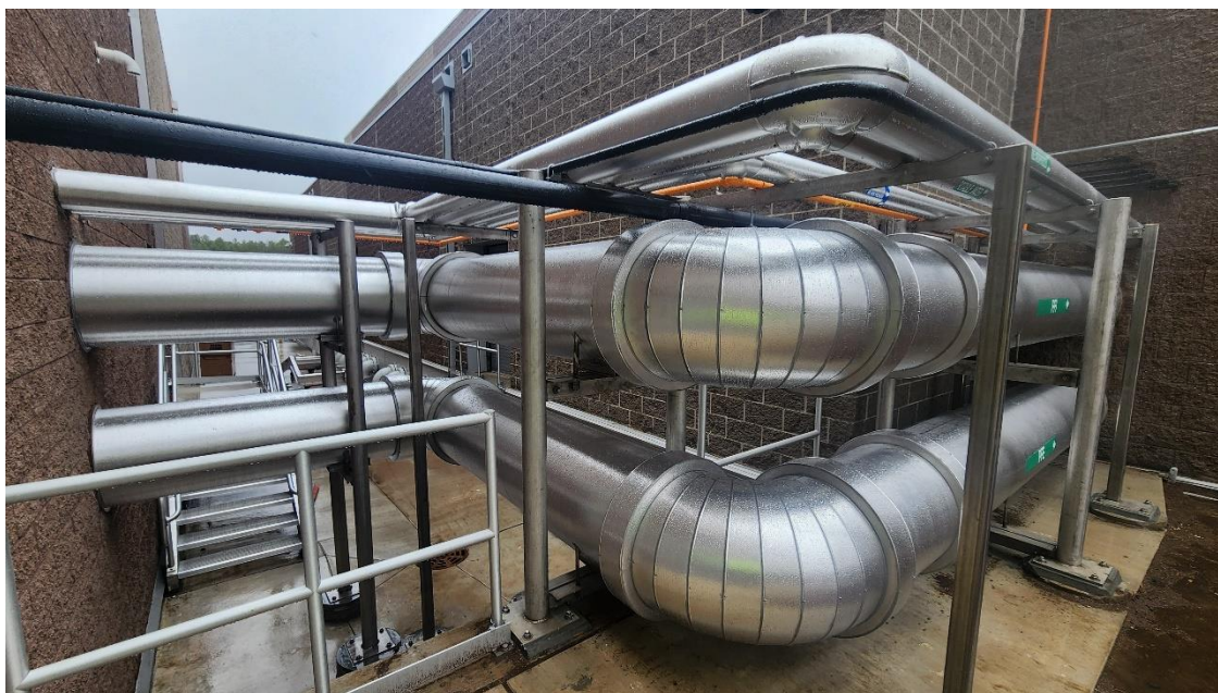
Insulation and jacketing completed on all pipe runs between Structure 100 and Structure 120.
