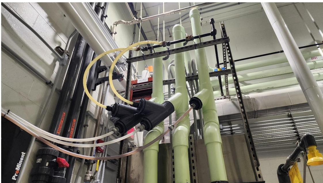
Heating water lines installed into carrier pipe for NaOH chemical feed lines to ensure lines don't freeze in Structure 100 (Process Building).
