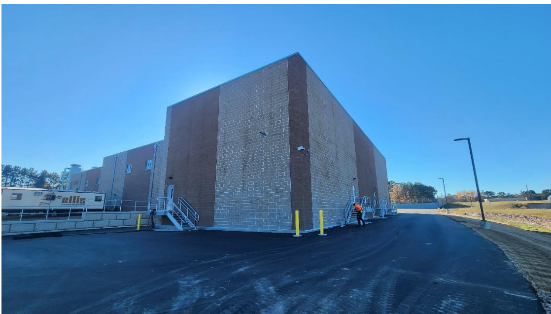
New asphalt and landscaping along north ditch of Structure 120 (PFAS Treatment Building).
