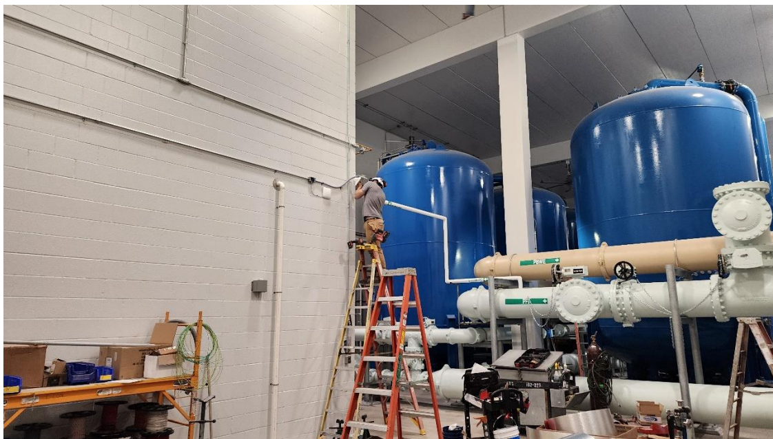
Interior security cameras and motion sensors installed in Structure 120.
