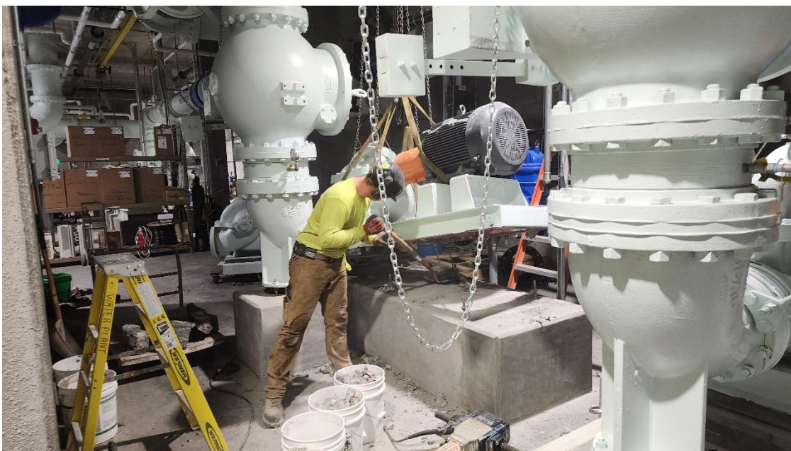
Demolition on third and final Filter Water Pump in Structure 100 (Process Building).
