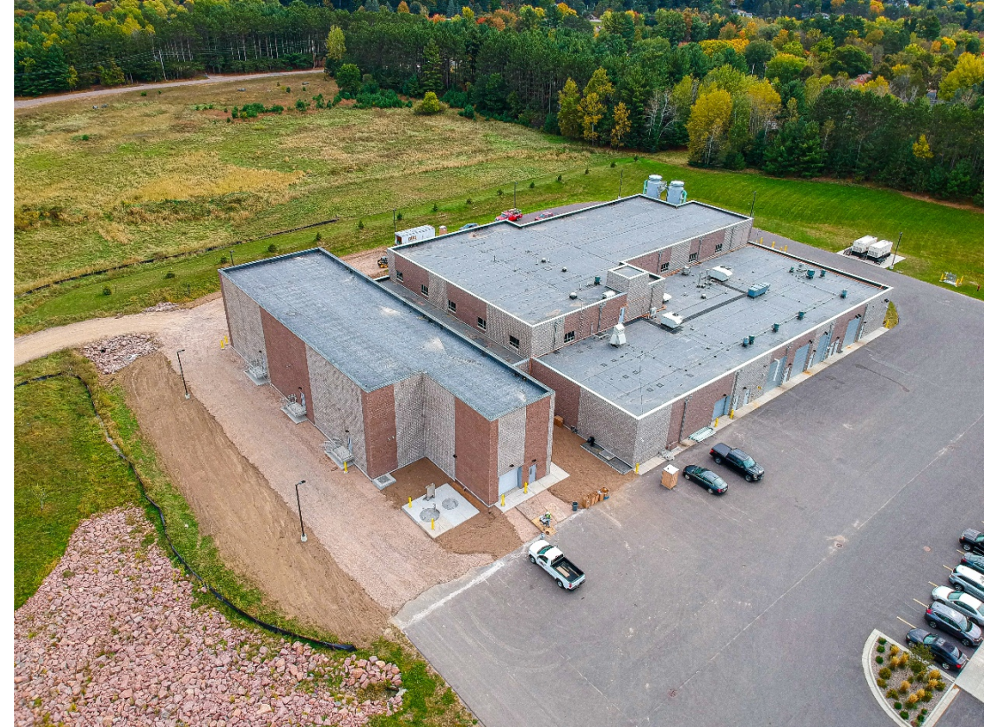
Aerial view of site, November 1, 2024. Note that paving and site work have been completed.
