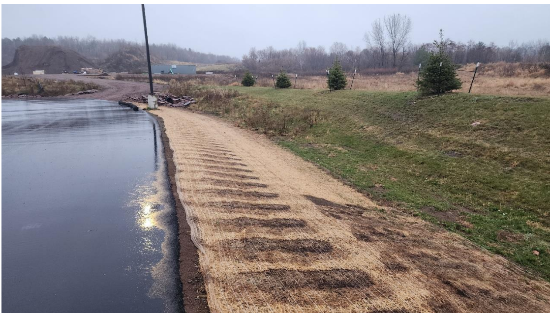
Landscape seed and mulch along east ditch east of Structure 100 and Structure 120.
