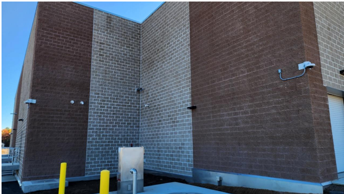
Exterior security cameras installed around Structure 120 (PFAS Treatment Building).
