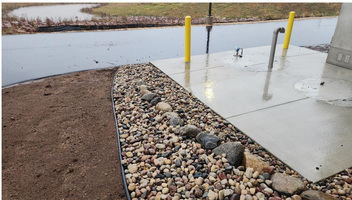
Landscape stone complete around MH410 and northwest side of Structure 120 (PFAS Treatment Building).
