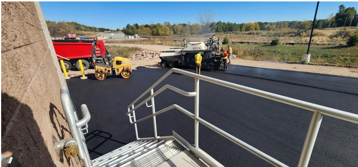
Asphalt being placed around Structure 120 (PFAS Treatment Building).
