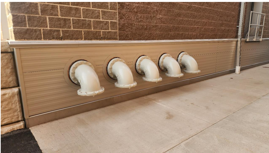
New wall panel is up on the northwall of Structure 100 between Structure 100 and Structure 120.
