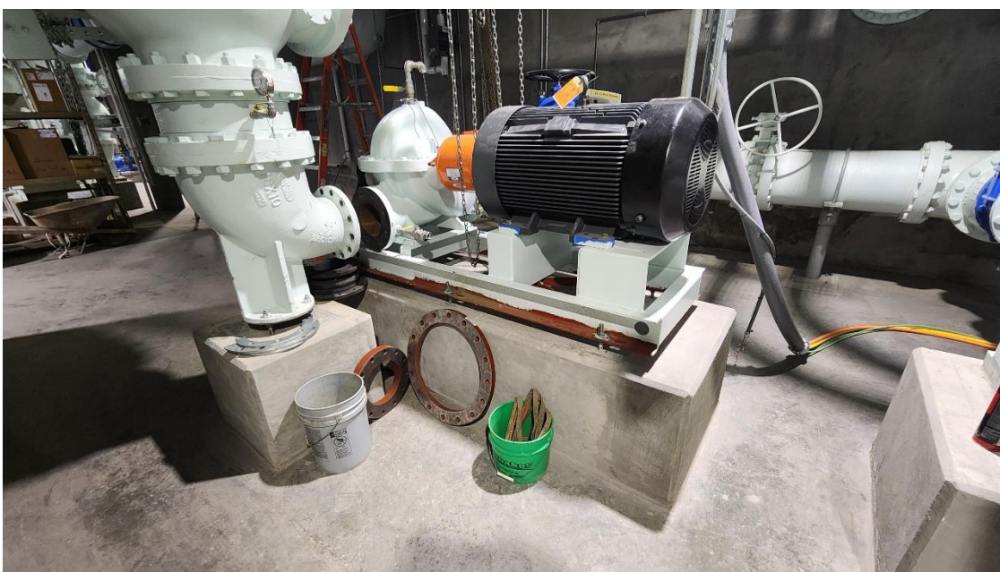
New Filtered Water Pump 0911 being set in place in Structure 100 (Process Building).
