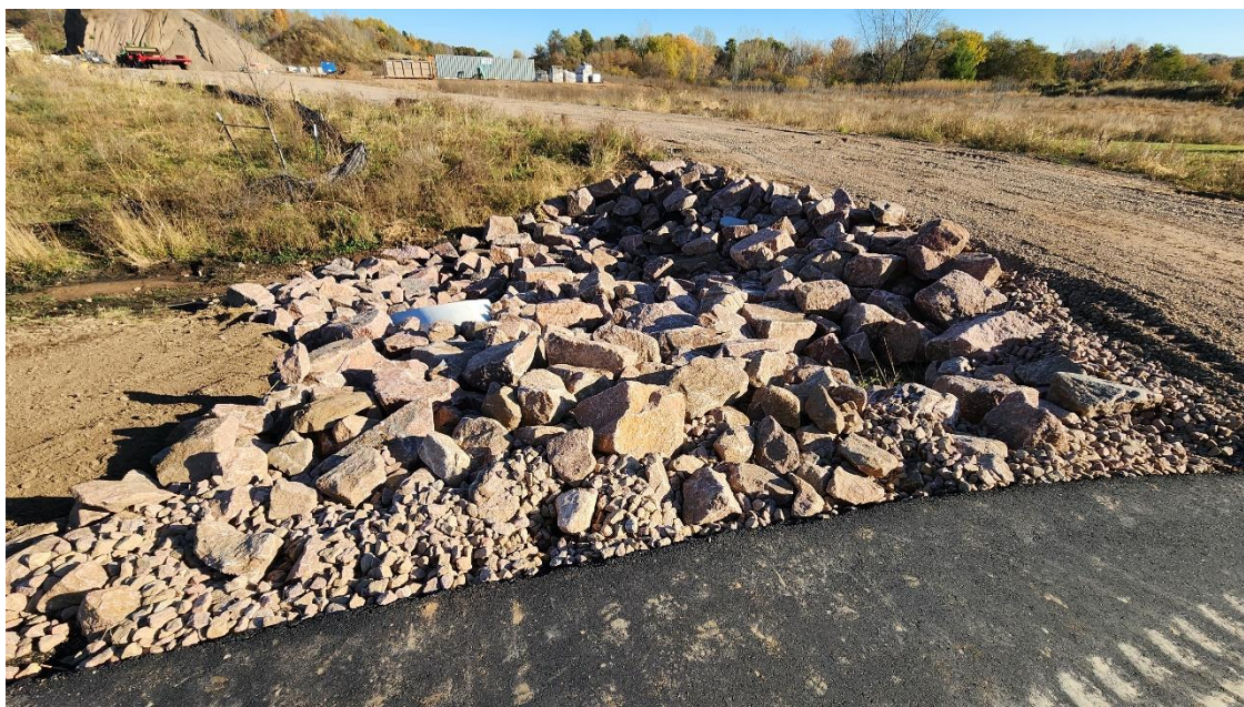
Rip rap placed on north and south sides of new temporary road at the NE side of Structure 120.
