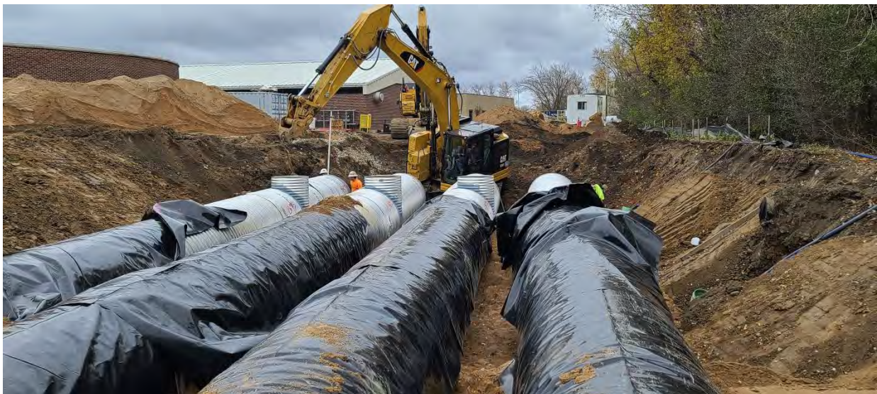
Installation of the storm water detention system on the east side of the site.
