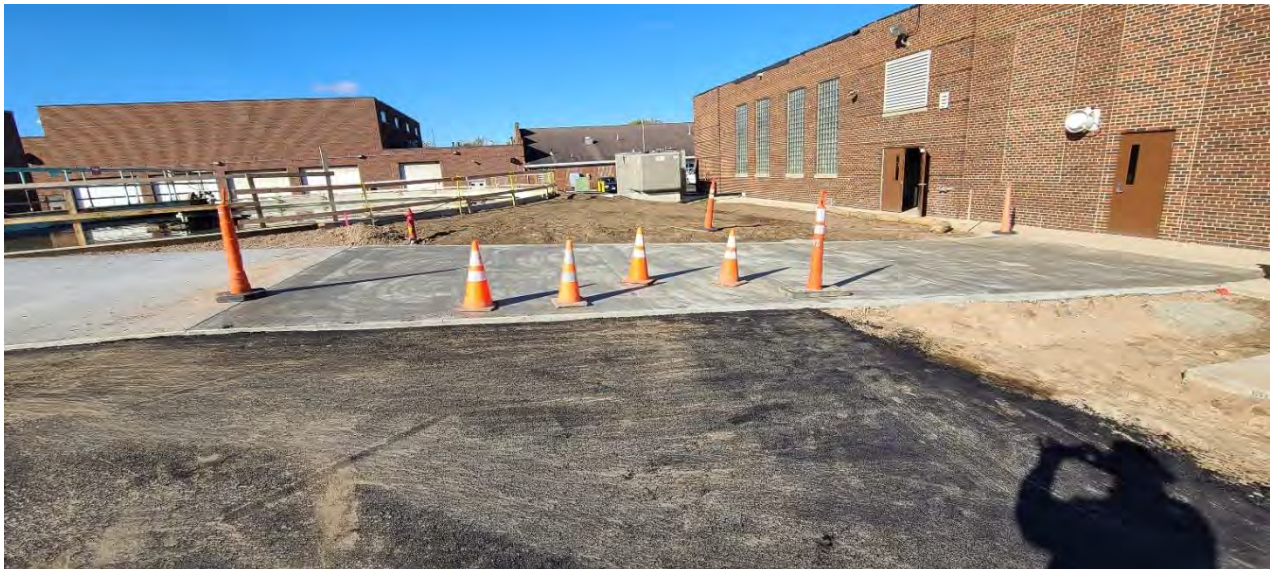
South side of Structure 100 (Main Building): concrete sidewalk placed over the top of the 900 Tunnel, asphalt binder has also been placed.
