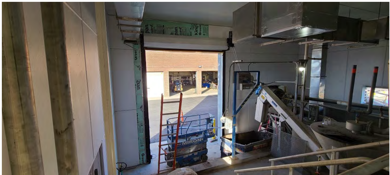
Structure 200 (Grit Building): new overhead garage door placed and progressing toward completion of interior fiberglass reinforced panels.
