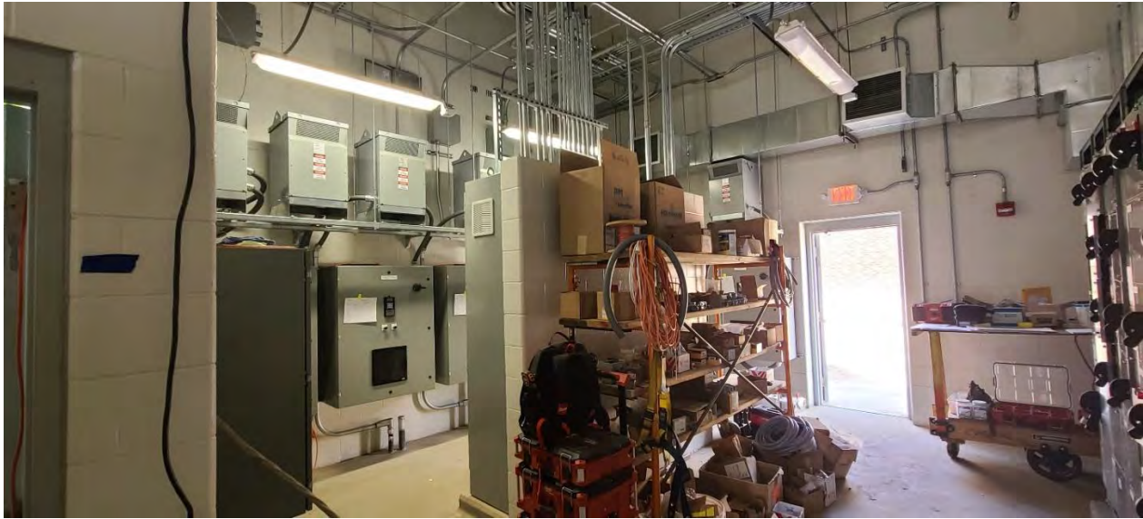
New electrical room and equipment for wiring Structure 610 (Chemical Building).
