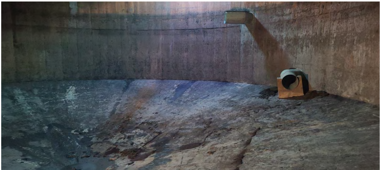
Interior of the cleaned Structure 710 (Digester1) waiting for new pipe
