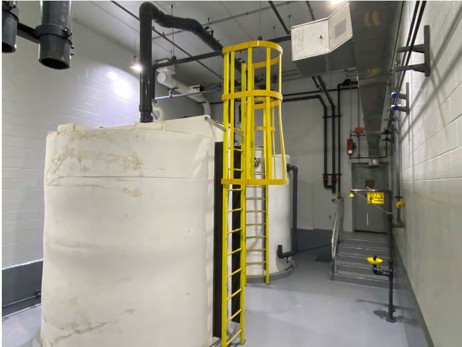
Chemical Storage Room – Floor Coating Complete
