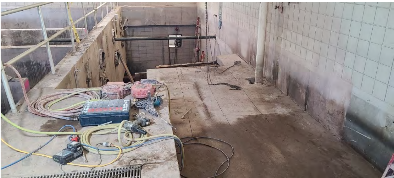
Concrete demolition work continues in the old sand filter area of Structure 600 (Effluent Building).
