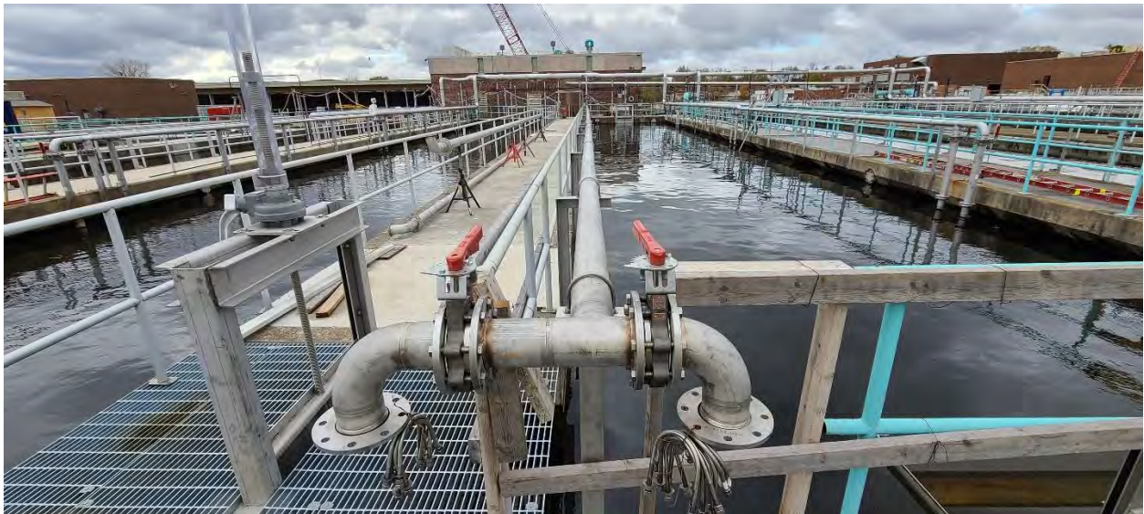
Structure 410 (Activated Sludge Basins): filled south aeration basins and the new 4-inch aeration header pipe and valves.
