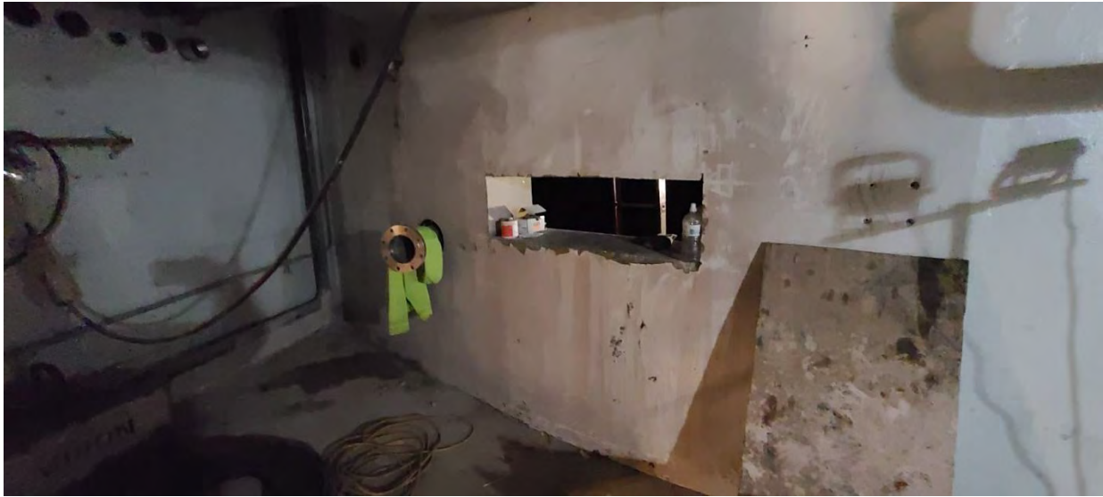
August Winters removing old piping out of tank wall for Structure 710 (Digester 1).
