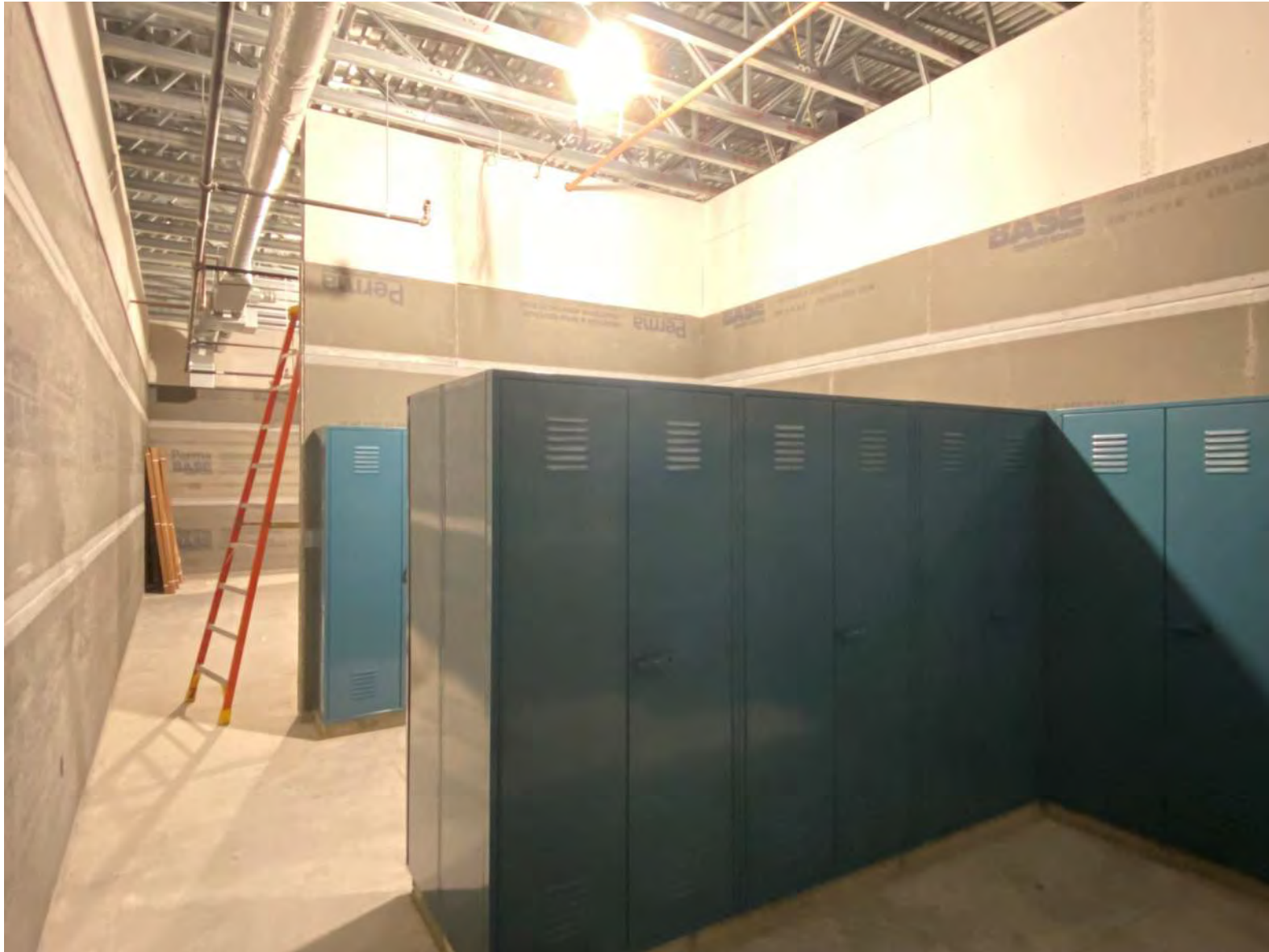
Lockers in Administration / Vehicle Storage Building
