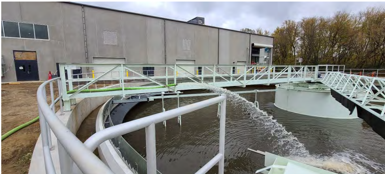
Filling Structure 540 (Secondary Clarifier 4) with W3 water.
