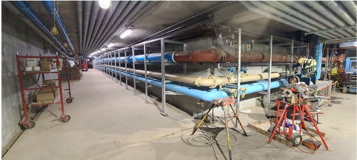
New lighting placed in Tunnel 910.
