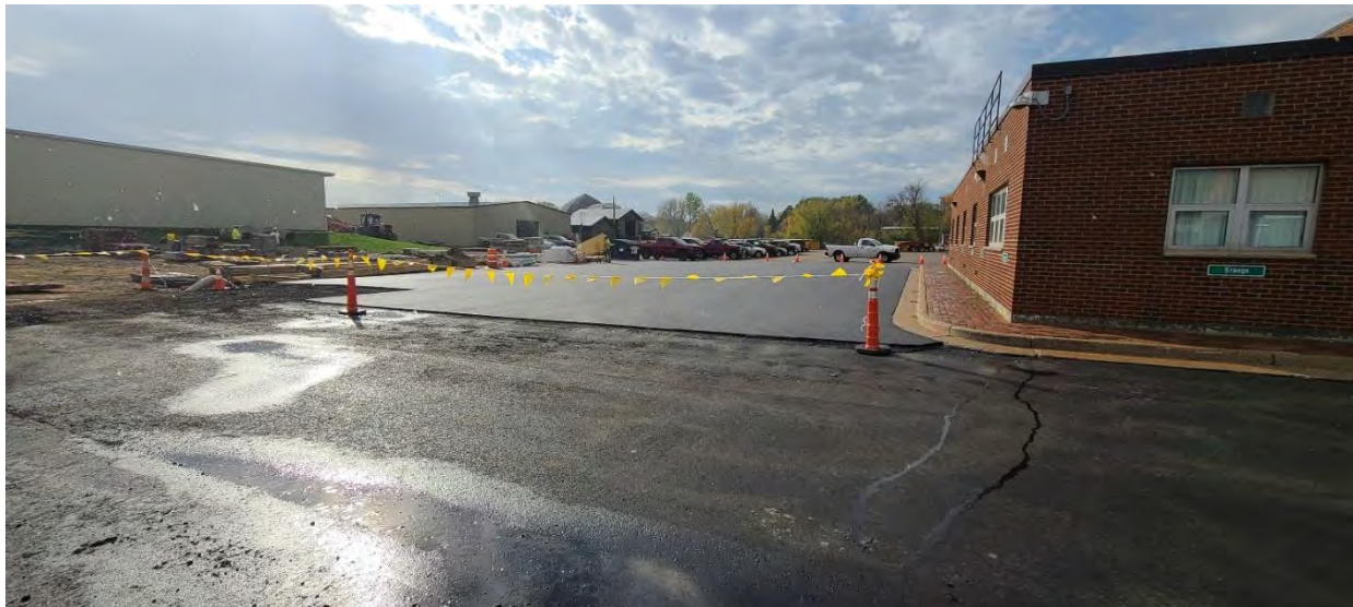
Surface and binder course placed at the north half of parking lot at Department of Public Works facility.
