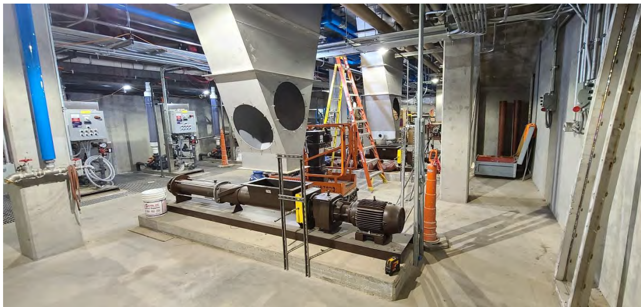
Structure 770 (Solids Building) TWAS Hopper and pump being placed waiting on parts and equipment.
