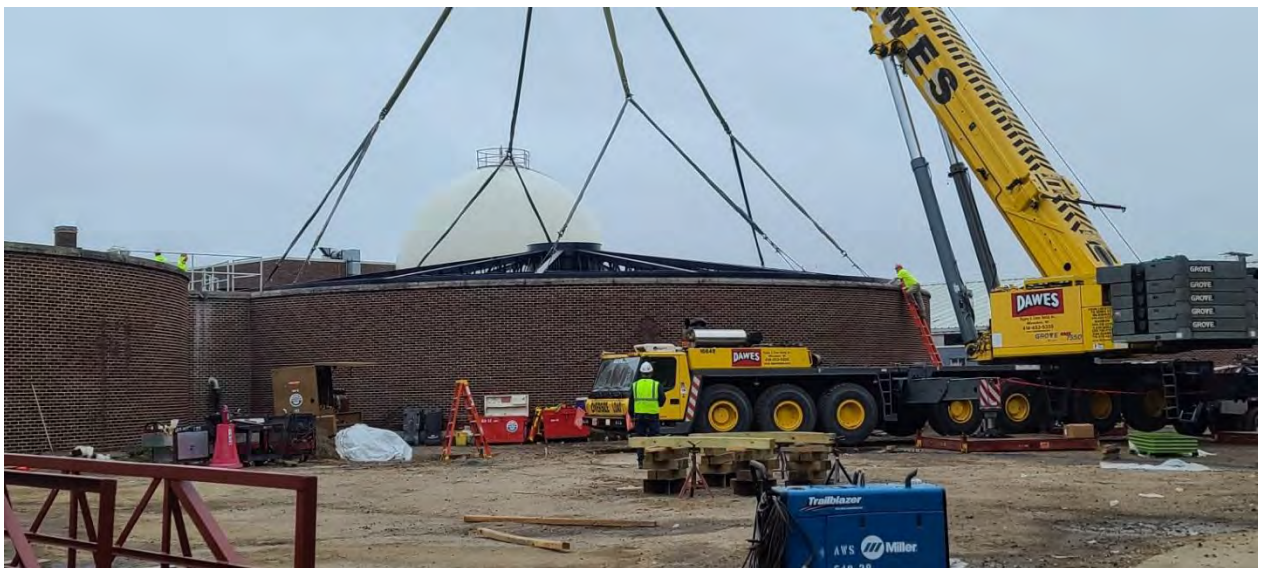
Placement of the Structure 720 (Digester 2) cover almost complete
