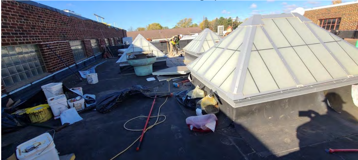
Roof demolition and work has been the started at Structure 100 (Main Building).
