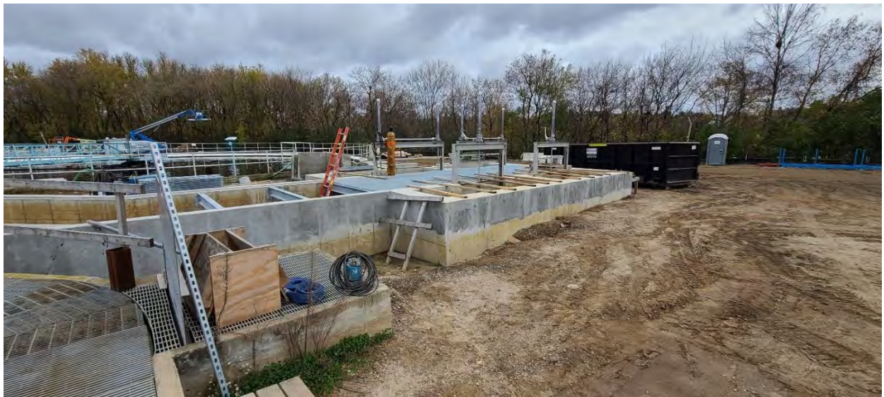
Structure 500 (Secondary Splitter) with new grating being placed.
