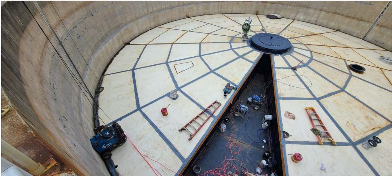
August Winters and Omni completing the internal and top side work on the new Structure 720 (Digester 2) cover.
