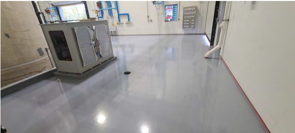
Concrete floor coated in chemical room of Structure 770 (Solids Building).
