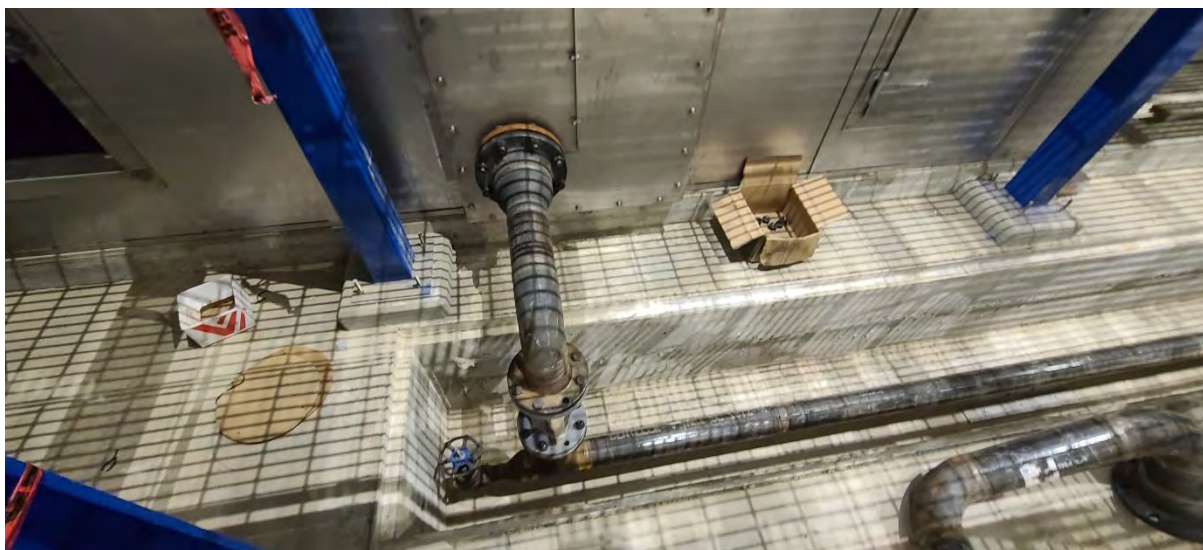
Thermal oil piping being placed in pipe gallery trench of Structure 770 (Solids Building).
