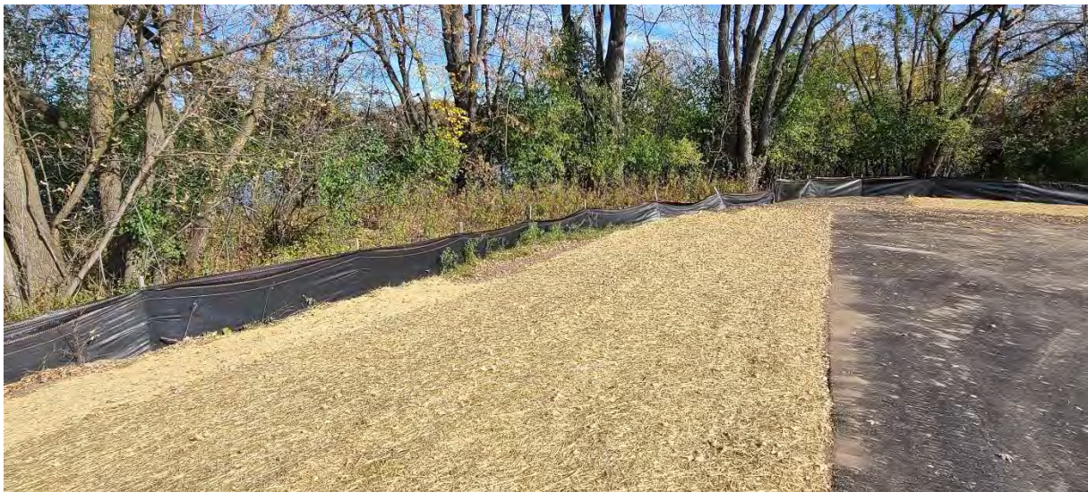
Grading, mulch and seeding around the paved areas of Structure 120 (Administration Building) has started.
