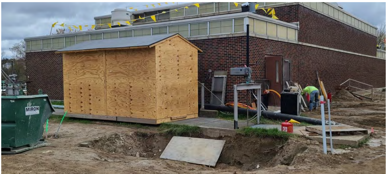
The temporary effluent flowmeter dog house has been completed and waiting on Effluent Flow Monitoring equipment to be installed
