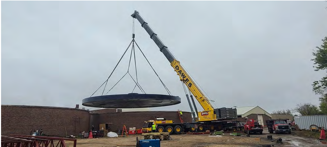
Lifting new Structure 720 (Digester 2) cover.
