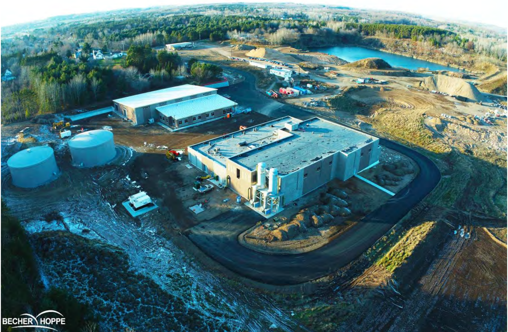
Site – looking Northwest
