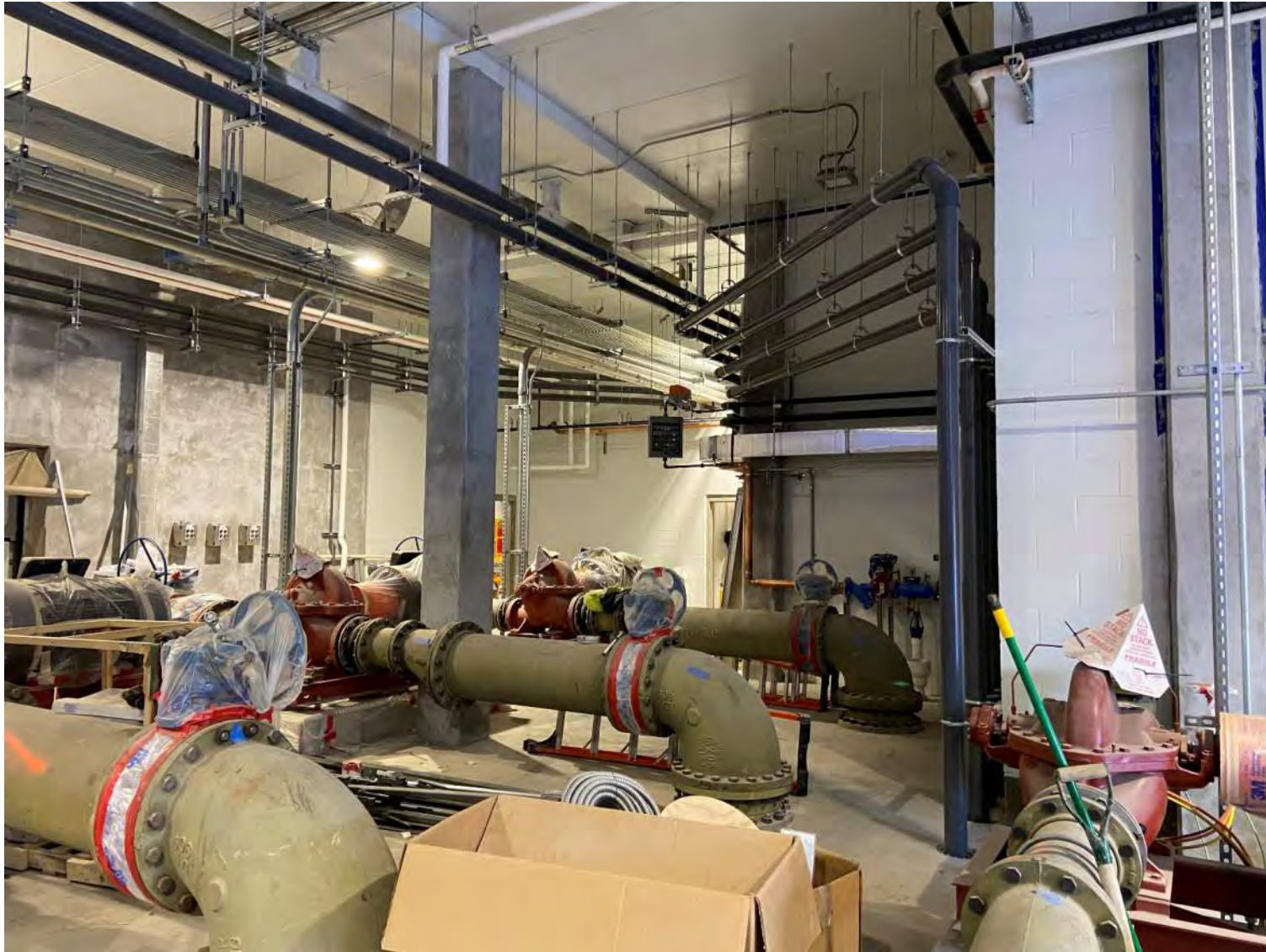
High Service Pump Area – Prepping for painting
