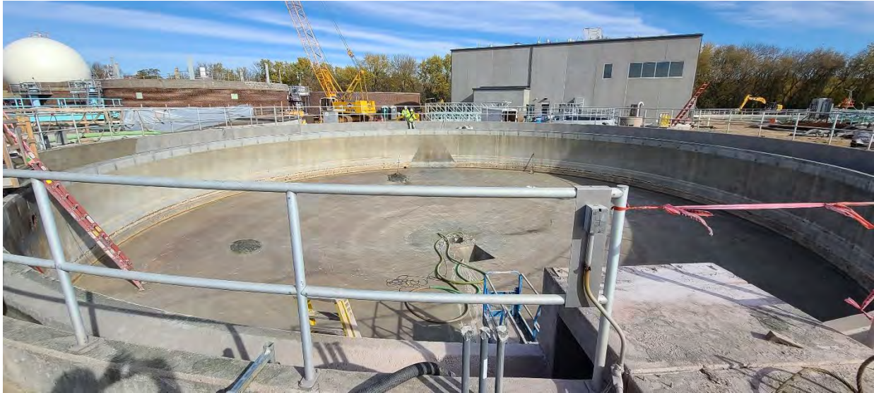
Removal of the existing mechanical equipment complete in Structure 340 (Primary Clarifier 4) and Omni prepping trough for coating
