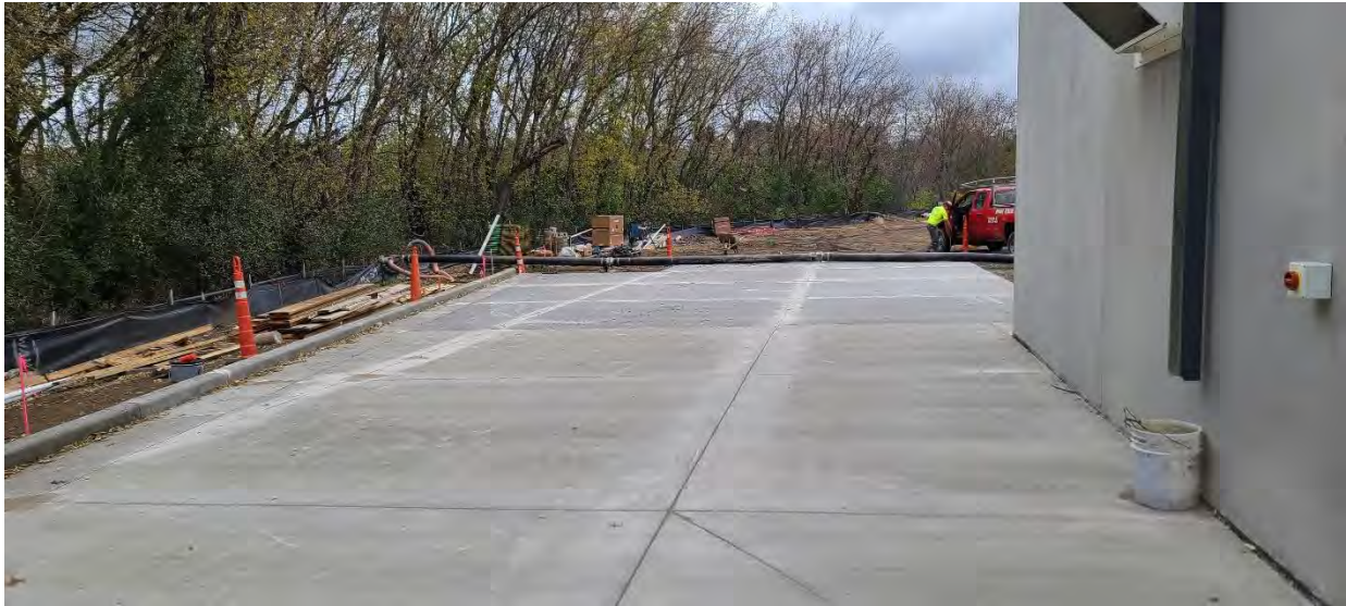
Placement of pavement around the east and northeast sides of Structure 770 (Solids Building) has started.
