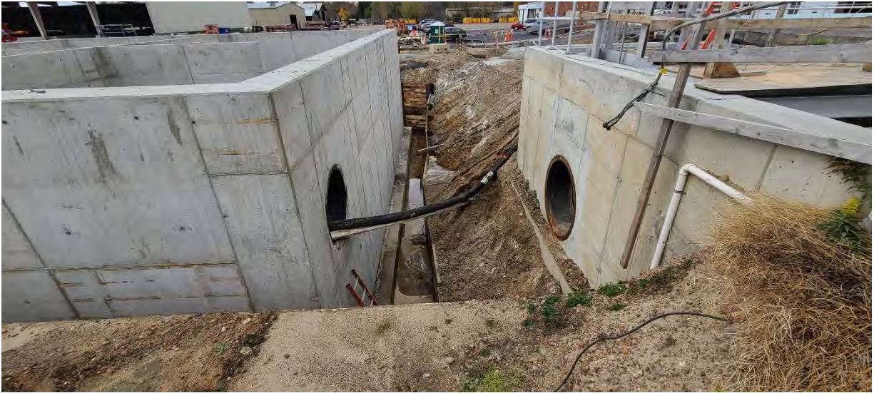
Foundation and concrete walls have been completed for the Structure 405 (Anoxic Selector Tank).
