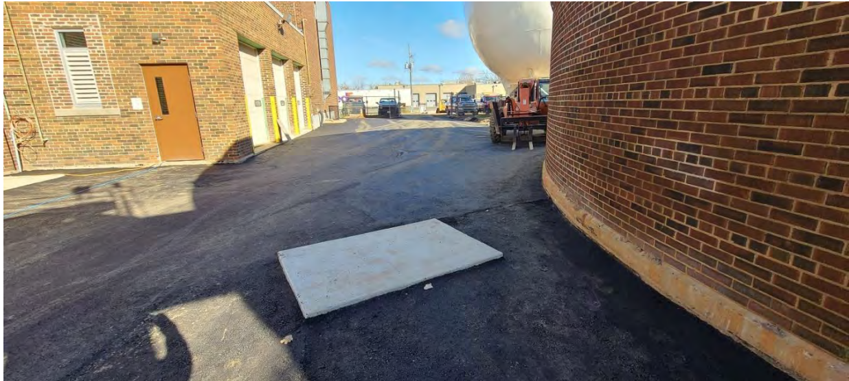
Asphalt binder course has been placed between the side walk for Structure 100 (Main Building) to the gas ball.
