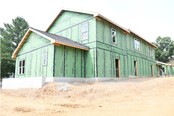
Photo 7 South & East Elevations
