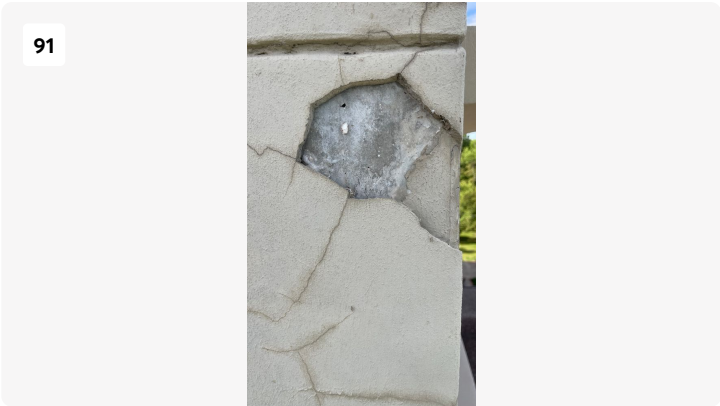
Review column for plaster slash cement covering, and then look at the coating that's adjacent to the concrete column.
