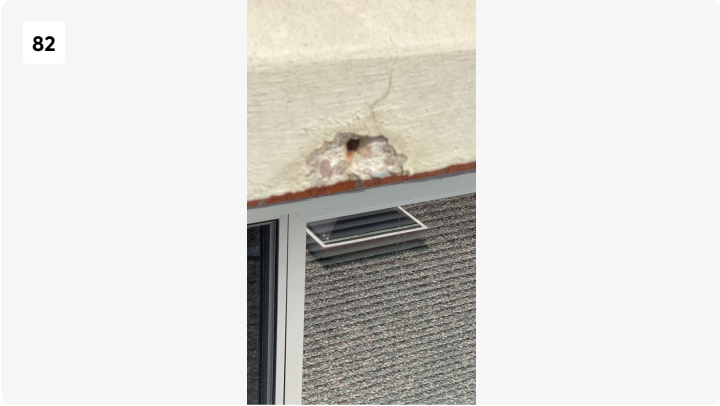
Project: Riverview Towers, LLC Date: Jun 2, 2026, 3:27 PM Creator: Melody Hamlin
