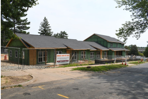
Photo 1 North & West Elevations
