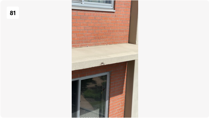
Project: Riverview Towers, LLC Date: Jun 2, 2026, 3:26 PM Creator: Melody Hamlin
