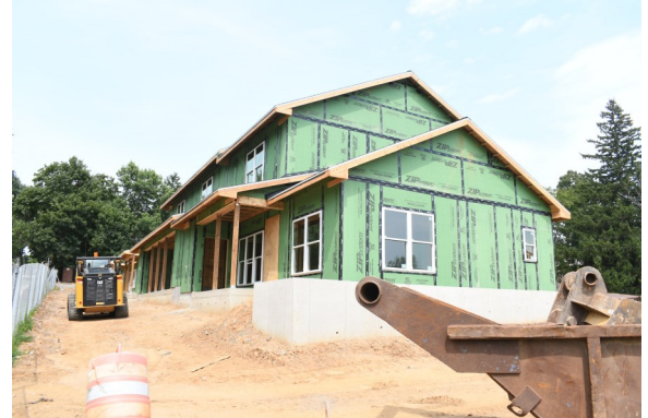
Photo 8 South & West Elevations
