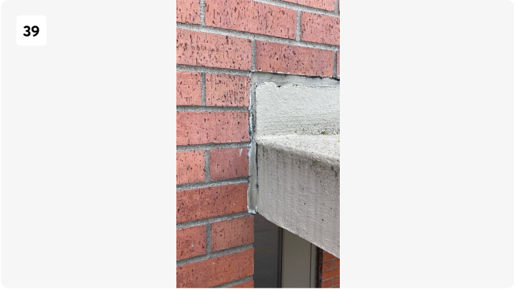
Project: Riverview Towers, LLC Date: Jun 1, 2026, 2:23 PM Creator: Melody Hamlin
