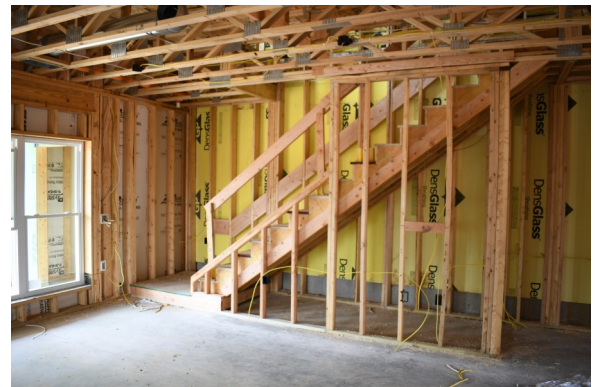
Photo 28 Unit F Living & Stair
