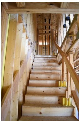
Photo 29 Unit F Stair
