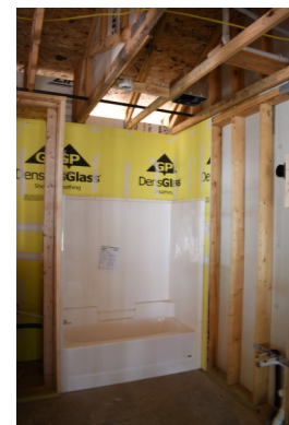
Photo 18 Unit A Bathroom
