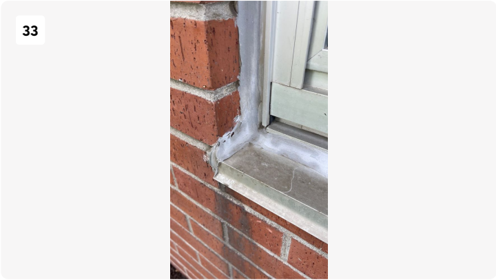
Project: Riverview Towers, LLC Date: Jun 1, 2026, 2:01 PM Creator: Melody Hamlin
