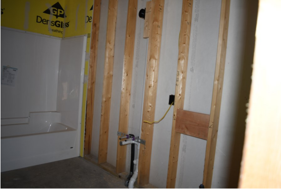
Photo 19 Unit A Bathroom
