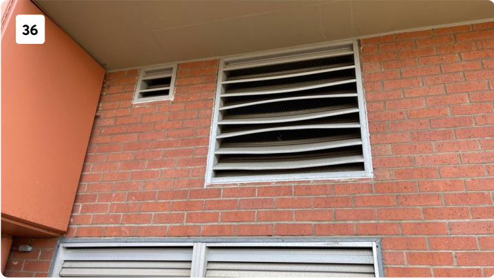
Project: Riverview Towers, LLC Date: Jun 1, 2026, 2:15 PM Creator: Melody Hamlin
