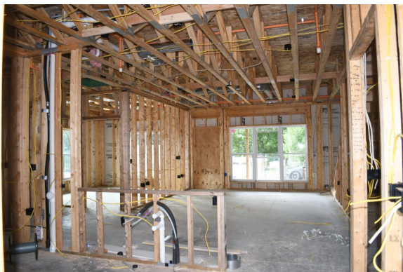
Photo 23 Unit F Kitchen & Living
