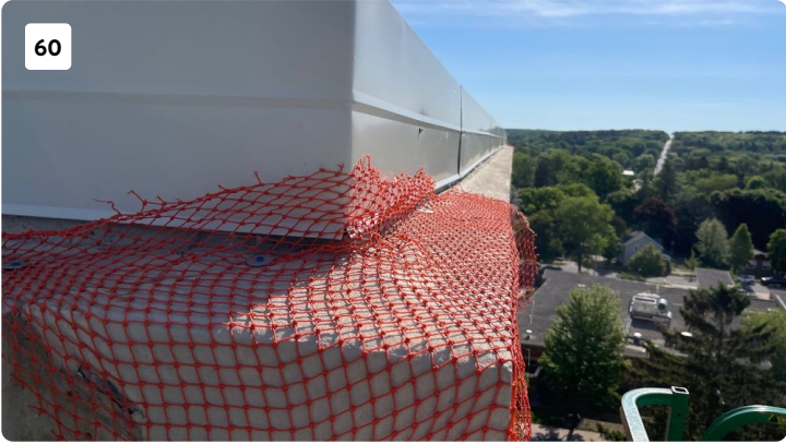
Southwest corner before starting south elevation
