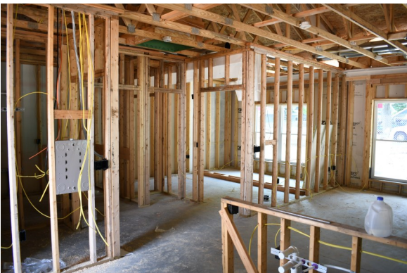
Photo 15 Unit A Mech & Bedroom
