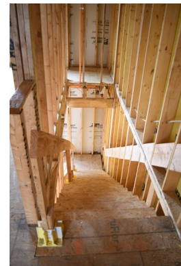
Photo 34 Unit F Stair
