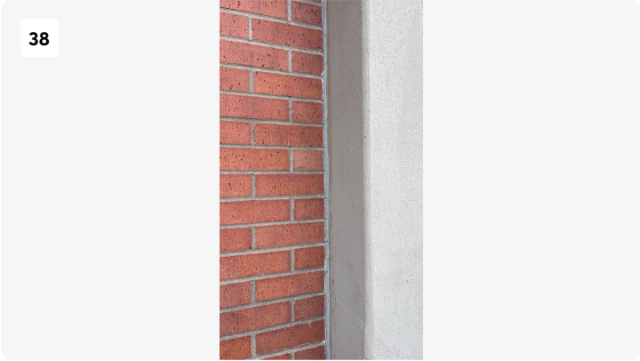
North 1st Floor interior joint of column
