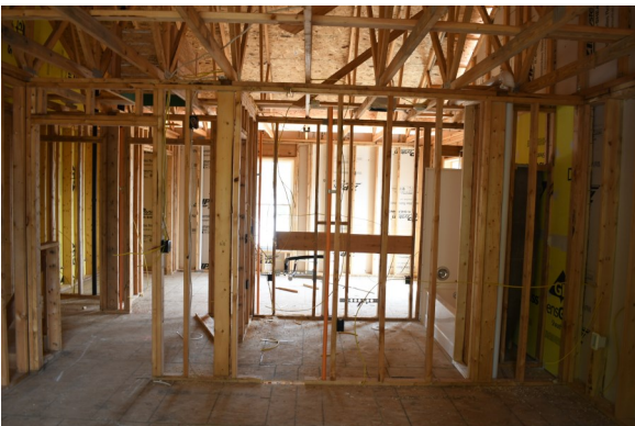
Photo 33 Unit F Bed 2
