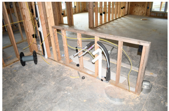
Photo 24 Unit F Kitchen
