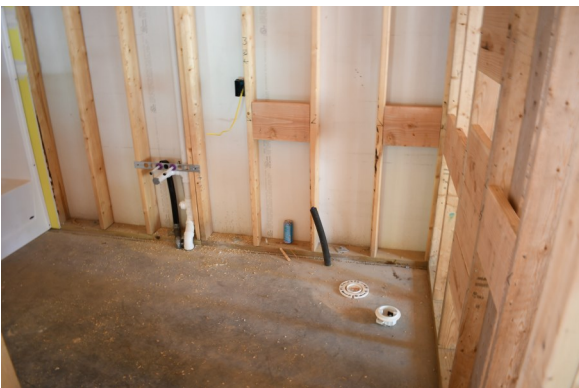
Photo 17 Unit A Bathroom
